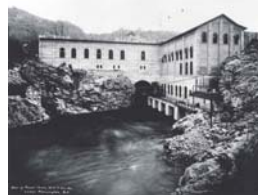
Rear of Lower Bonnington power house - W.K.P. & L. Co.
